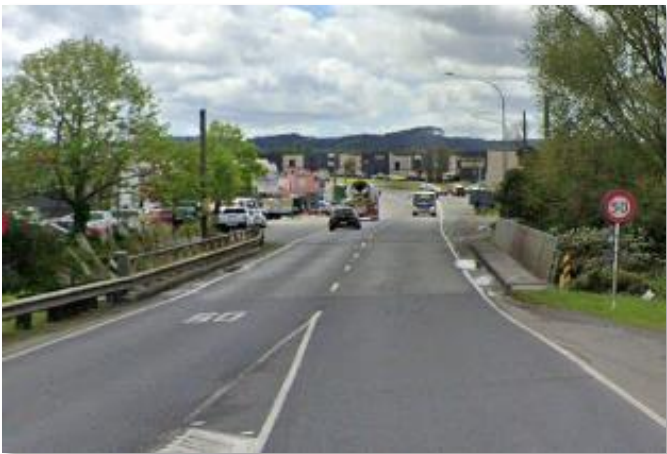
Constrained two-lane bridge over the Hingaia Stream
