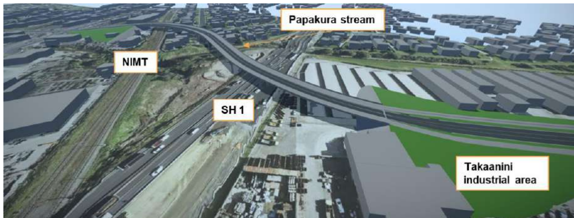
Figure 5-2 : South IBC Rangi Road Viaduct Recommendation
