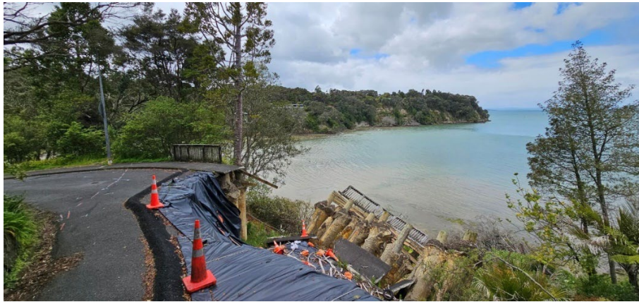
Large Slip on the corner of Paturoa Road, previous retaining wall has failed and slipped towards the beach.
