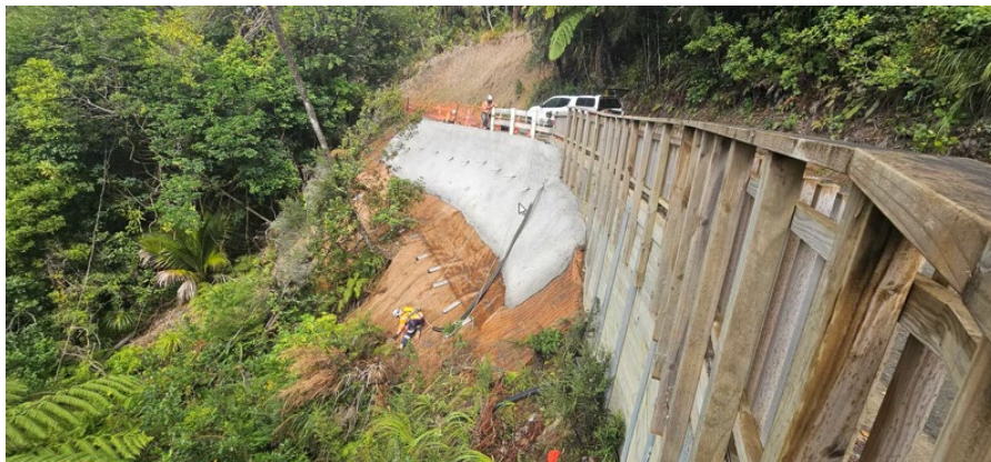
Progress photos in March of the slip repair on Whatipu Road.
