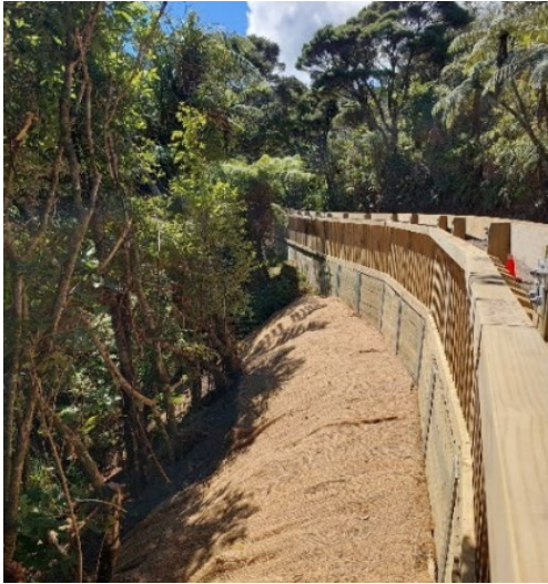
Slip site RP2.5 Lone Kauri Road, works started 15 January 2025. The handrail in the photo is above a retaining wall built prior to the cyclone. The retaining wall will be extended either side of this location.
