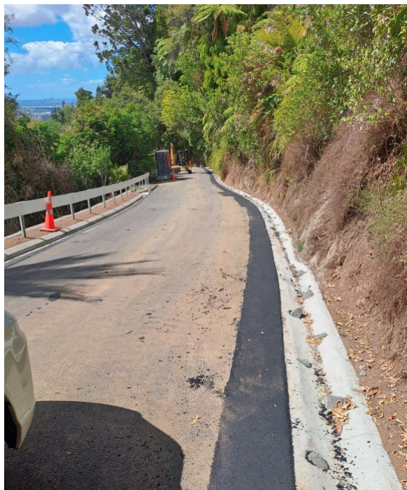
Site RP1.318 Mountain Road completed
