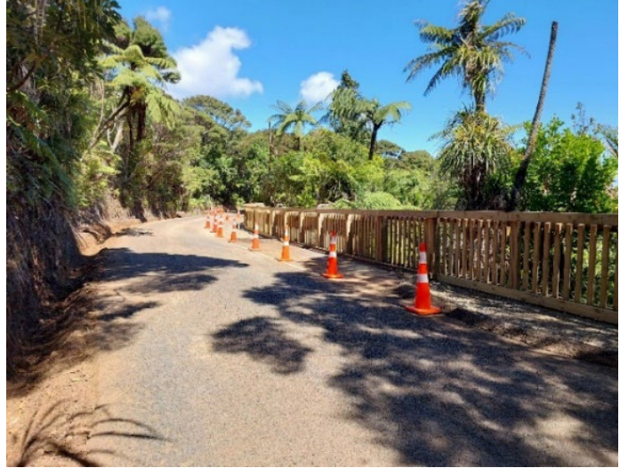
Slip site RP2.5 Lone Kauri Road, works started 15 January 2025. The handrail in the photo is above a retaining wall built prior to the cyclone. The retaining wall will be extended either side of this location.
