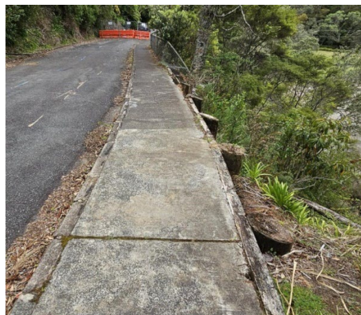
Large Slip on the corner of Paturoa Road, previous retaining wall has failed and fallen towards the beach.
