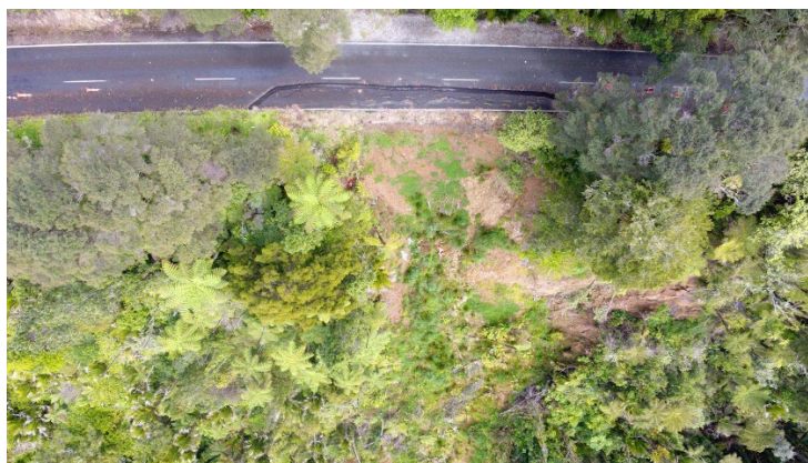
A view of the slip from above before the works started.
