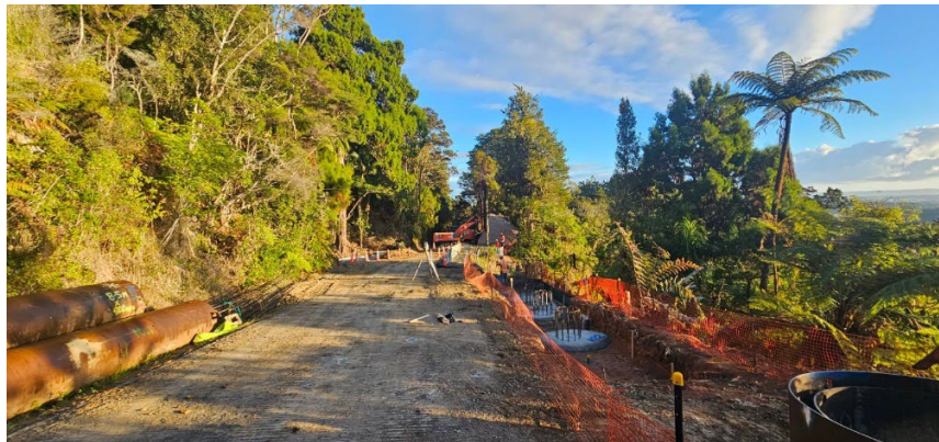
Works underway on-site
