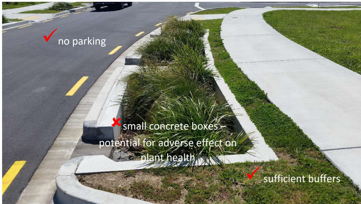
FIGURE 5-5: CONCRETE BOX RAINGARDEN (2)
