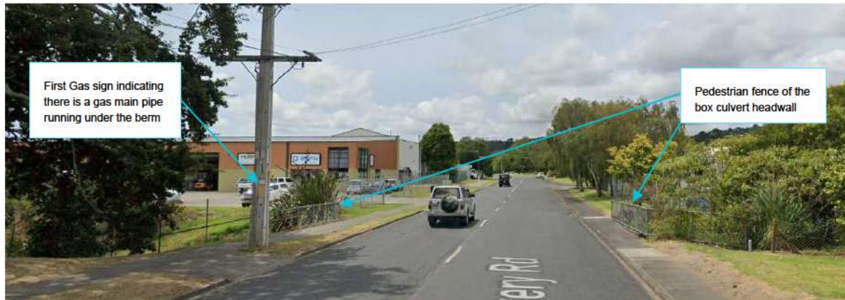
Figure 3 Croskery Road Box Culvert that crosses Otuwairoa Stream/ Slippery Creek
