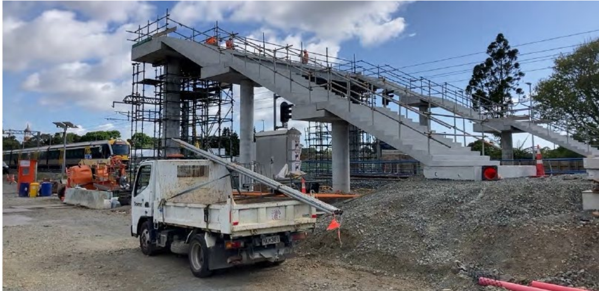
New overbridge at Middlemore Station
