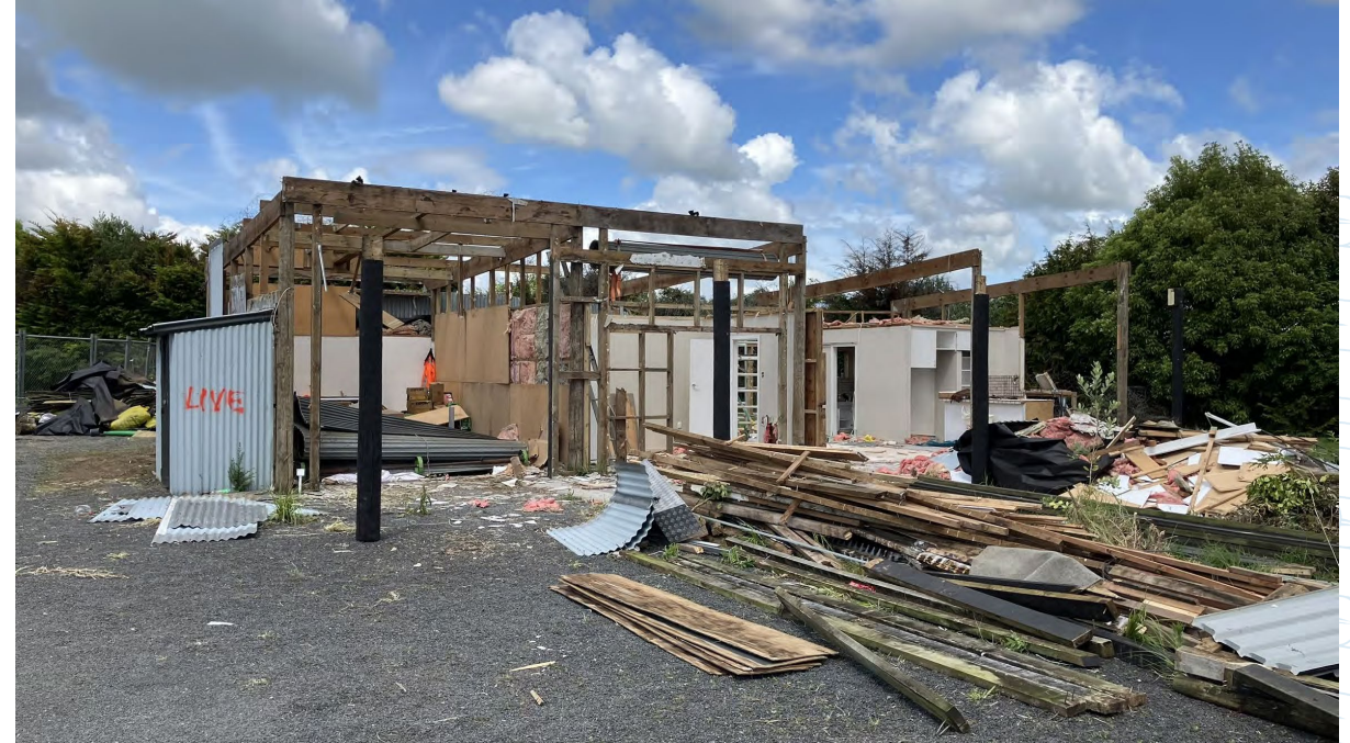
Sustainable demolition at Drury Station – building demolished and rebuilt with all original items in Northland
