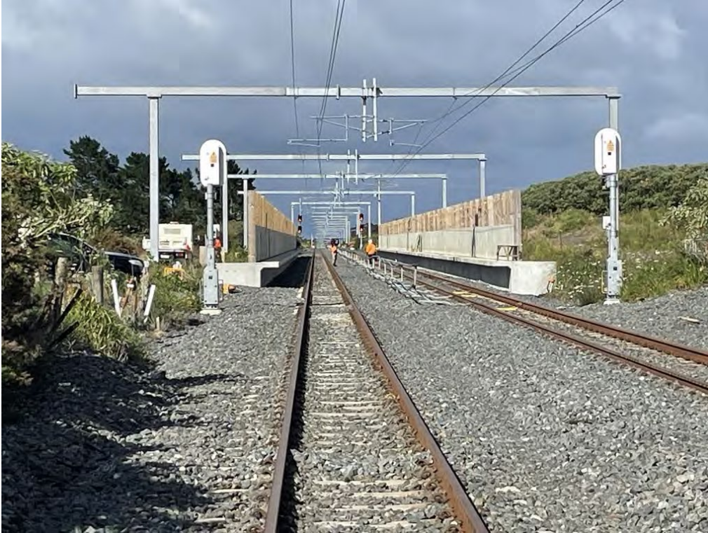
Platform faces built at Ngākōroa Station
