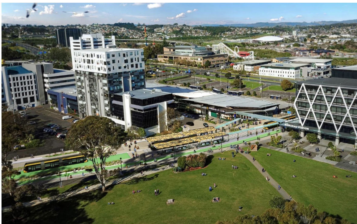
Figure 15-4: A2B rapid transit at Manukau station
