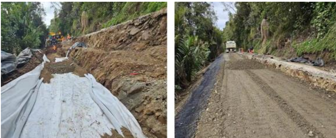
Back fill almost completed.
