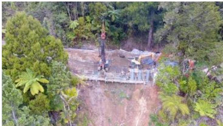
The drilling underway in May.
