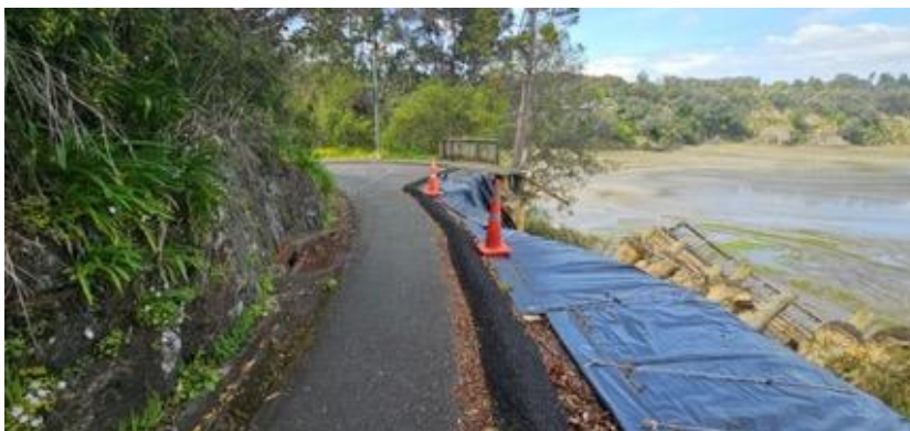
Large Slip on the corner of Paturoa Road, previous retaining wall has failed and fallen towards the beach.
