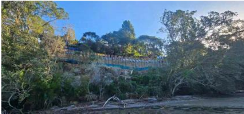
Paturoa Road - The new timber retaining wall.
