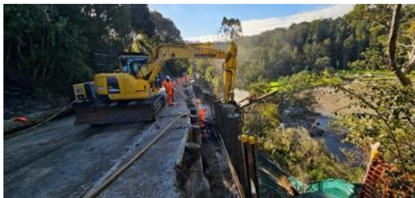
Paturoa Road - Anchors being installed through the new retaining wall.
