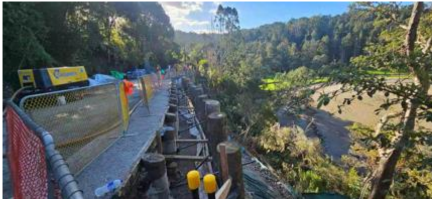
Paturoa Road - A view from below. Anchors being installed in the new wall.
