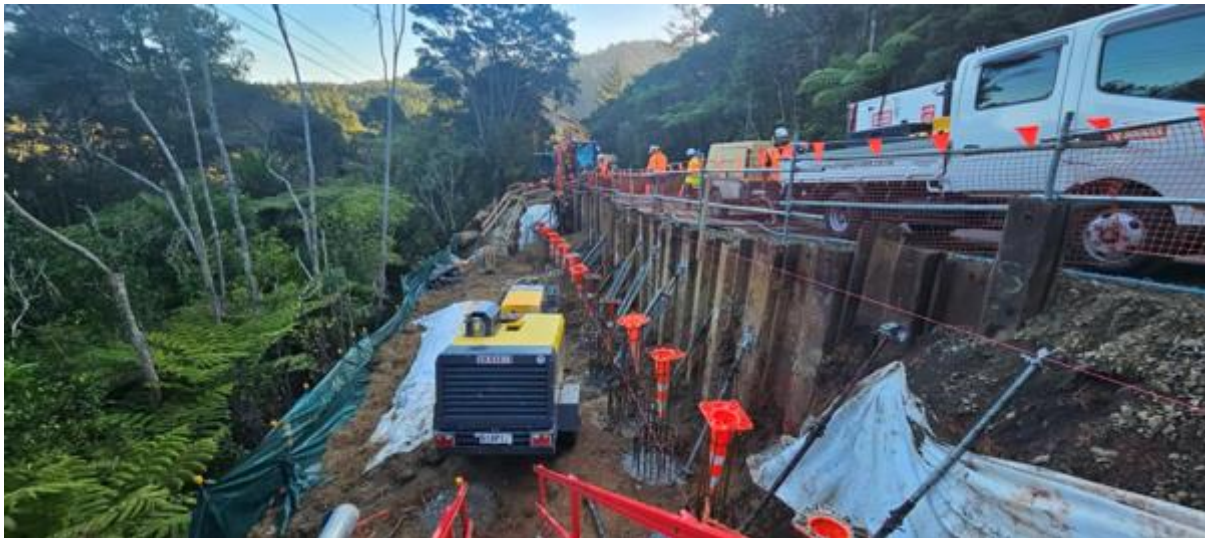
Site RP11.327 Huia Road, works underway, sheet pile wall is installed to temporarily retain the road while the permanent wall is installed.
