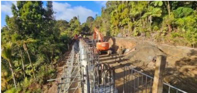
The final piles are installed.
