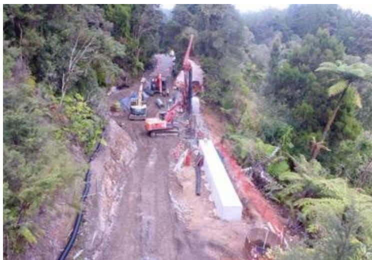
A side on view of the site.
