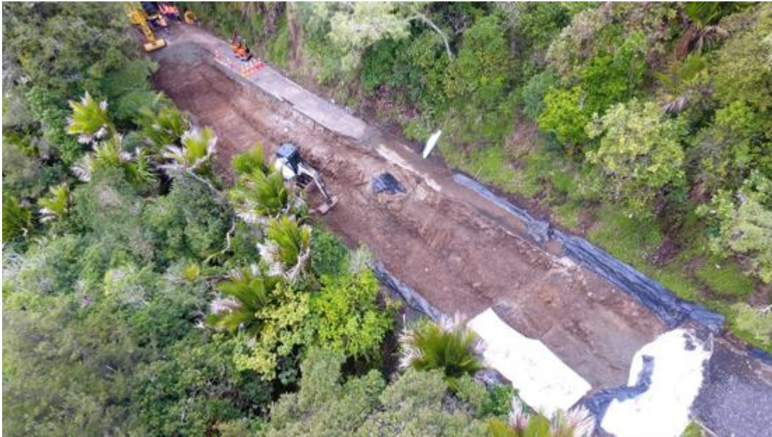
The excavation underway.
